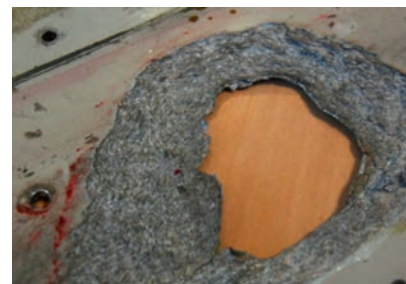
Figure 3 Example of galvanic corrosion of a galley storage container caused by a well known brand of soft drink
