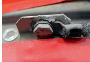
Figure 11 Corrosion of electrical bondings, vital for aircraft systems safety (lightening strike, static electricity discharge, etc), could cause them to become ineffective
