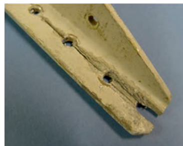
Figure 17 Stress induced corrosion along the fastener holes
