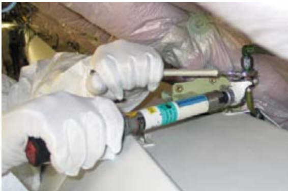
Figure 9 Use two wrenches during disconnec- tion/reconnec- tion of connectors and torque at right value
