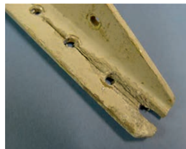
Figure 17 Stress induced corrosion along the fastener holes
