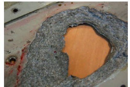
Figure 3 Example of galvanic corrosion of a galley storage container caused by a well known brand of soft drink
